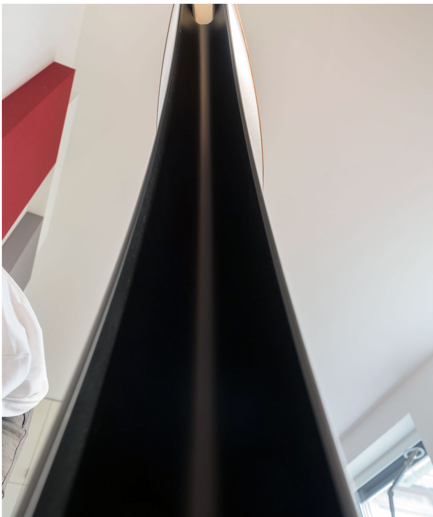
The back of the stalls: The perspective could be deceiving. The stands are not open to the rear, but closed with a concave counterpart to the outer shape. (Photo: F. Borowski)
